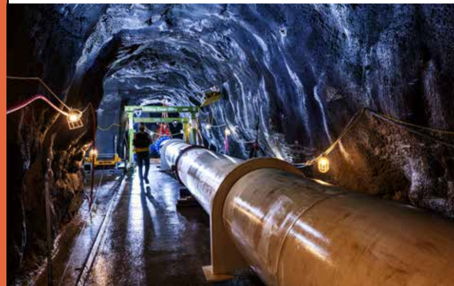
Installing a 36-inch conveyance pipe and a 24-inch guard valve at Culmback Dam.
