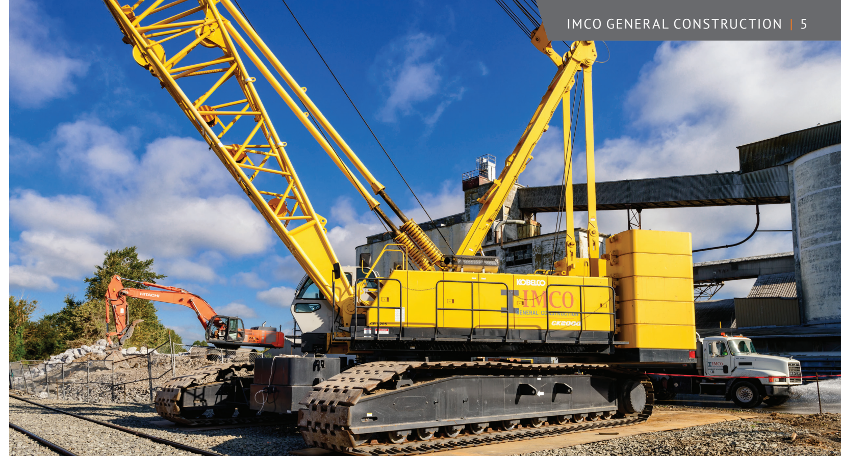
Picture above is from IMCO's BNSF slope stabilization project completed over the summer.
