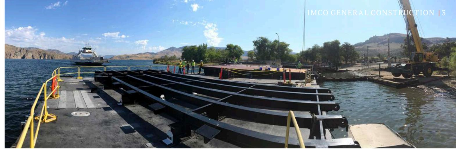
*Pictured above, IMCO begins the construction of the new ferry terminals at Lake Roosevelt with structural steel installation on top of the new pontoons.*
