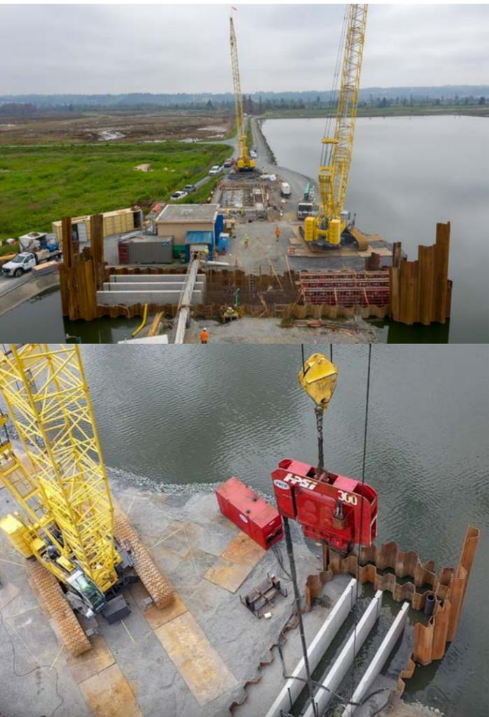
The sheet pile surrounding the newly constructed concrete culvert was removed earlier this summer. The cast-in-place culvert is now fully functional and in use. Adjacent to the culvert, IMCO is building a pile-supported chlorination building. The Slab on Grade was completed last week, and the CMU wall construction and structural steel erection are under way. Outfall excavation, manhole installation, and steel roof erection will happen later this summer.
