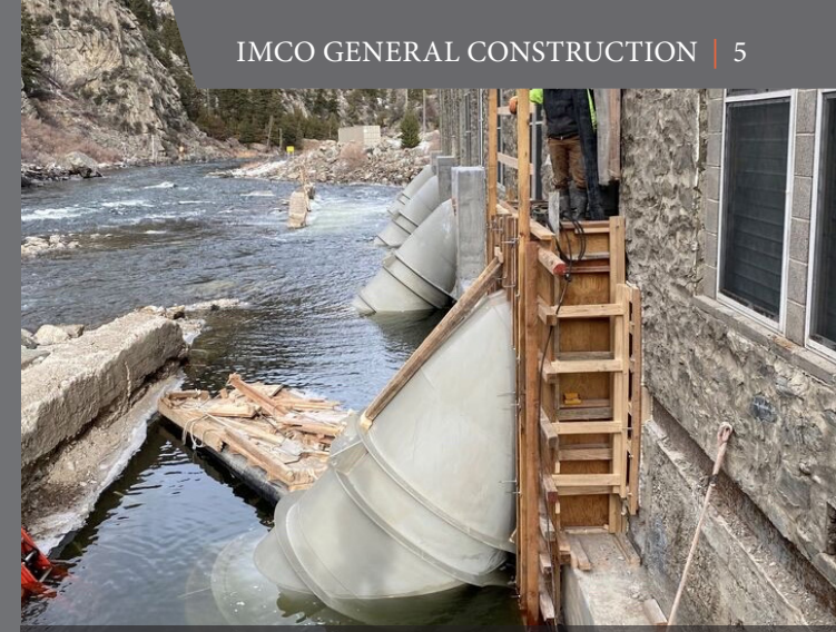
Tail race with new draft tubes installed at Madison.
