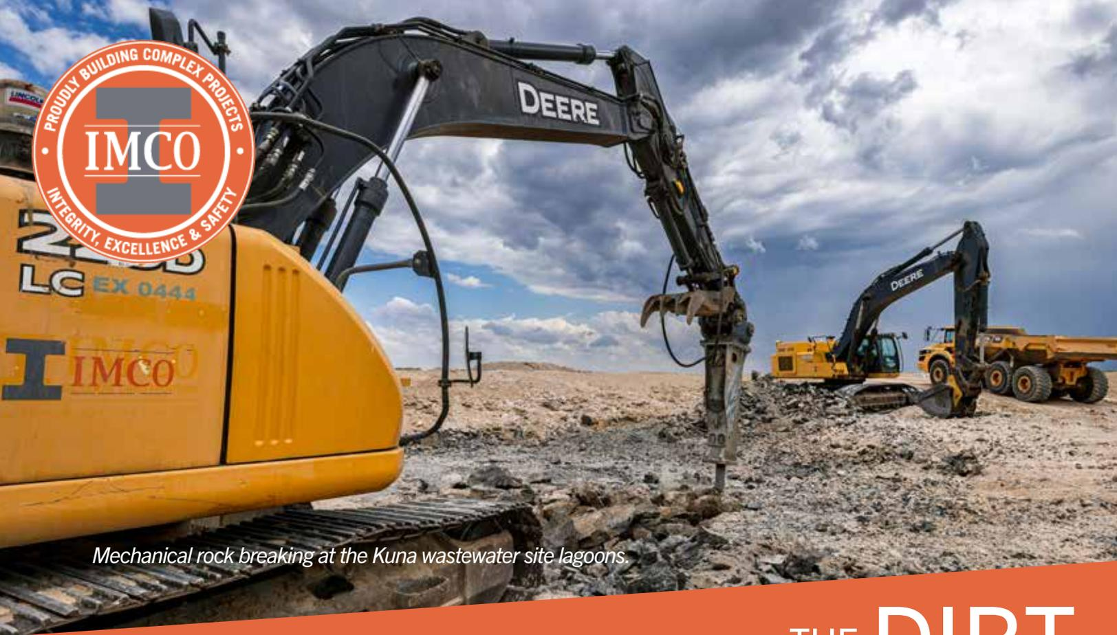
*Mechanical rock breaking at the Kuna wastewater site lagoons.*
