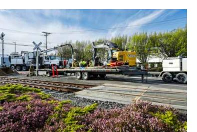
As the project moves into the final phase along Roeder Avenue, the focus will shift to construction on BNSF Railway property. This next stage will involve a trenchless crossing beneath the railroad tracks, installation of more than 2,000 lineal feet of welded HDPE pipe of various sizes, slip lining an existing sewer force main, and a final cutover from the existing sewer lift station.
