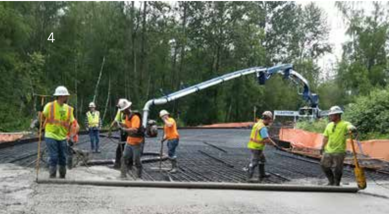
On June 14 th , crews poured 350 yards of concrete on East Maple Road (left).
