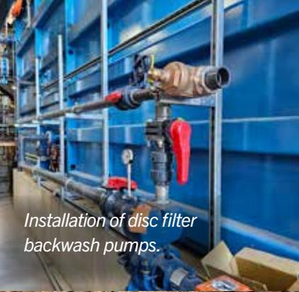
*Installation of disc filter backwash pumps.*
