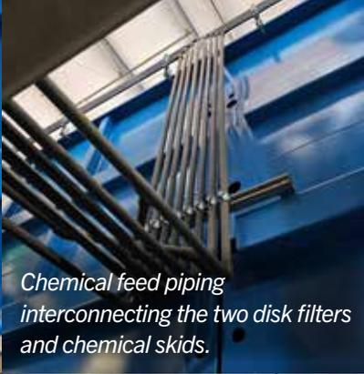
*Chemical feed piping interconnecting the two disk filters and chemical skids.*
