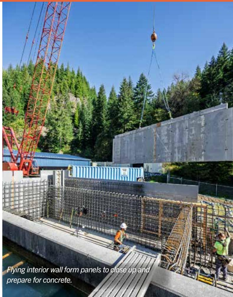
*Flying interior wall form panels to close up and prepare for concrete.*
