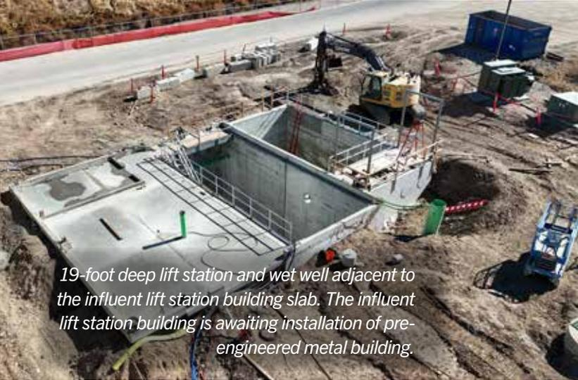
*19-foot deep lift station and wet well adjacent to the influent lift station building slab. The influent lift station building is awaiting installation of pre-engineered metal building.*
