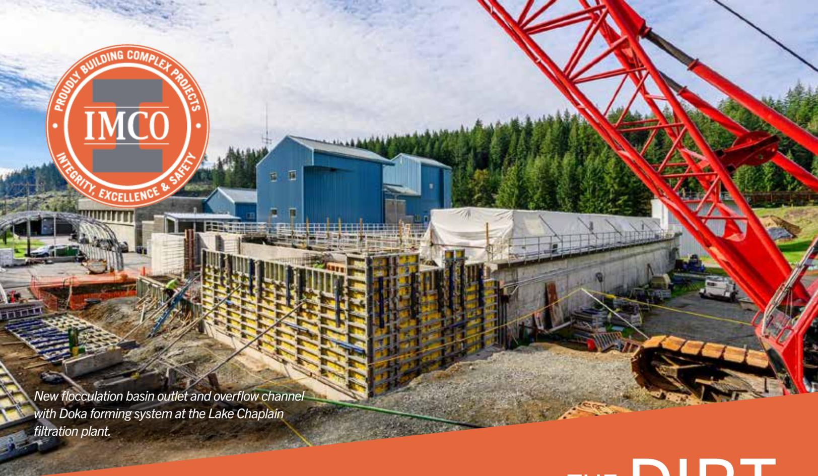
*New flocculation basin outlet and overflow channel with Doka forming system at the Lake Chaplain filtration plant.*
