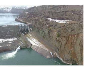
IMCO's Oxbow spillway team has launched the remediation project, a critical infrastructure initiative aimed at enhancing the long-term performance and reliability of the existing spillway at the Oxbow Dam. The project, commissioned to address recurring undercutting issues at the spillway toe, will significantly strengthen and extend the structure to improve safety and functionality.
