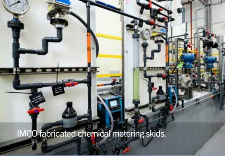
IMCO fabricated chemical metering skids.
