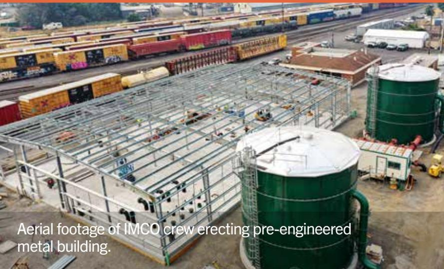
Aerial footage of IMCO crew erecting pre-engineered metal building.
